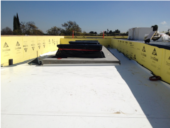
Date:02/19/16 Roofing installation at mechanical area adjacent to community room.
