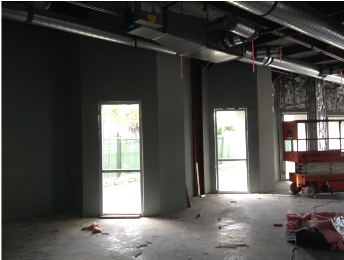
Date: 03/09/16 Drywall being installed along West elevation of Adult Collection Area.
