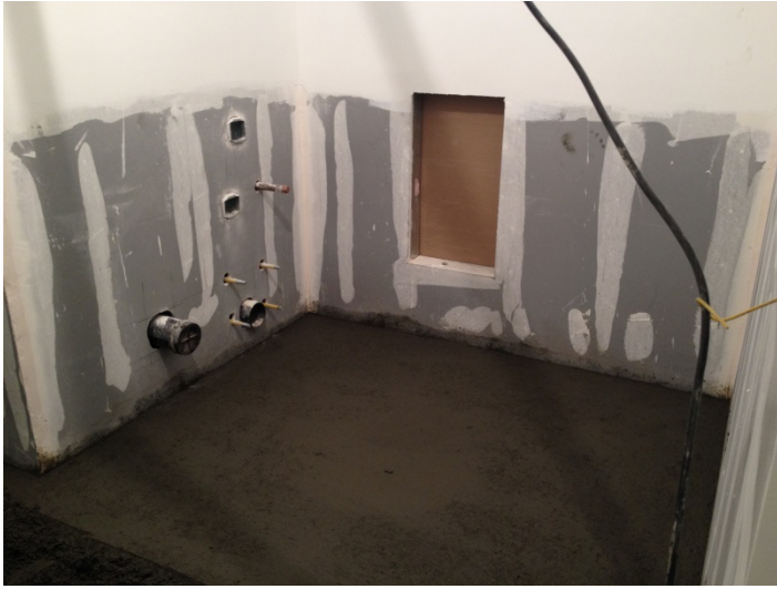
Date: 03/08/16 Staff restrooms being painted and being prepped for tile installation.
