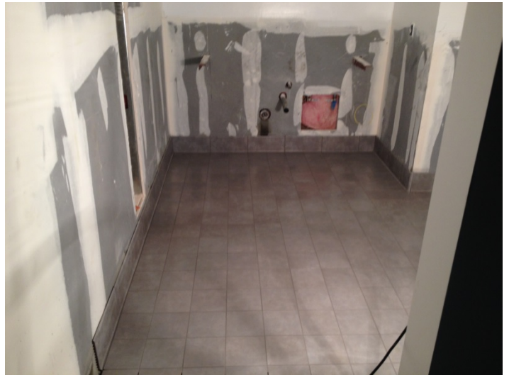
Date: 03/11/16 Tiling installed in staff restrooms.
