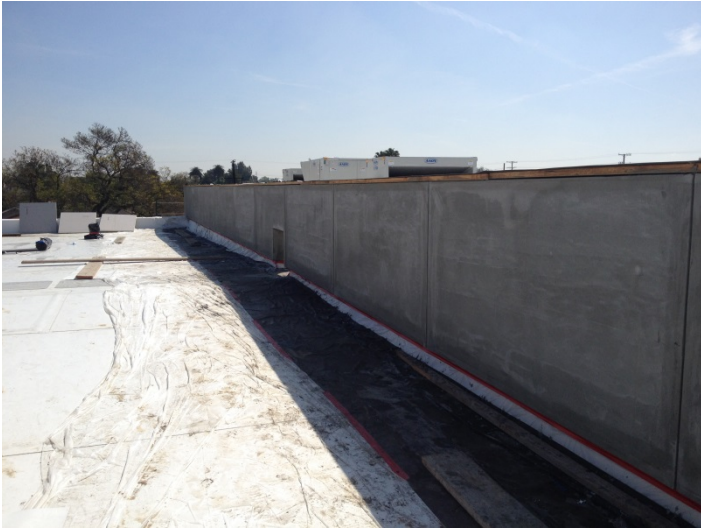
Date: 03/15/16 EIFS panel well North of Mechanical II with applied genesis DM.
