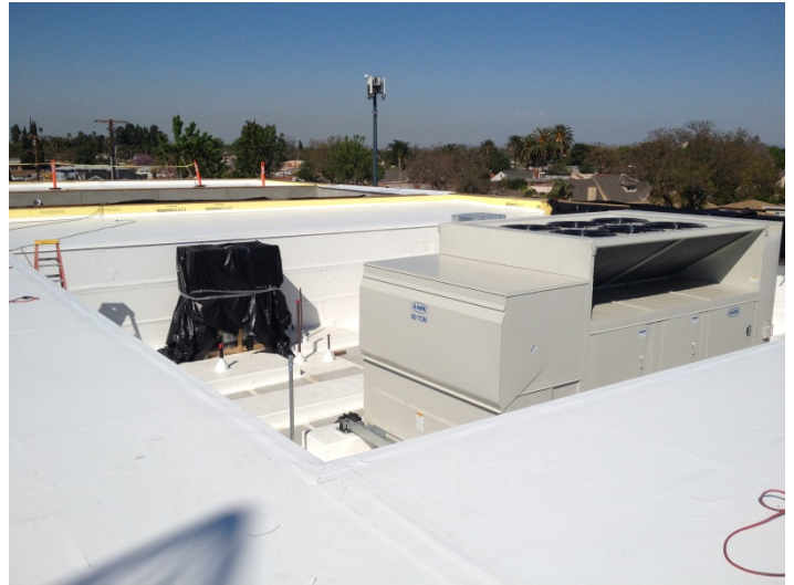
Date: 03/17/16 High roof adjacent to mechanical I, with sarnafil membrane installed.
