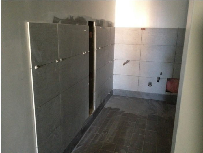
Date: 03/17/16 Wall tile installed in Staff restroom.
