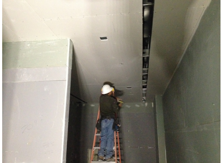
Date: 03/15/16 Gypsum board installed at ceilings inside the women's restroom.
