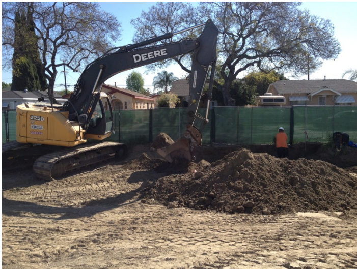
Date: 03/25/16 WCF excavating for site wall footings along the East end of the project site.
