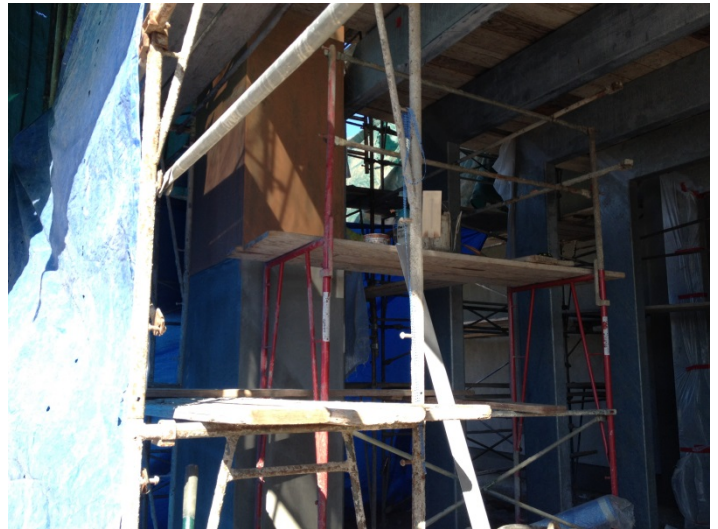
Date: 03/25/16 Column at entrance to Library with skim it product being applied in preparation for final finish.
