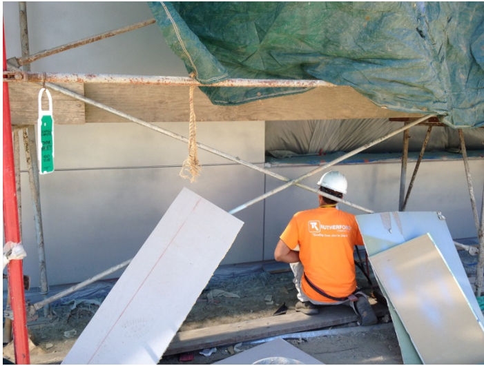
Date: 03/24/16 Rutherford spraying final metallic finish to EIFS located at East elevation, at the Family Learning Center.
