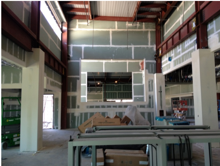
Date: 03/29/16 Progress of mudding and taping throughout the Library. Photo is of periodicals section, looking East from the adult collection area.
