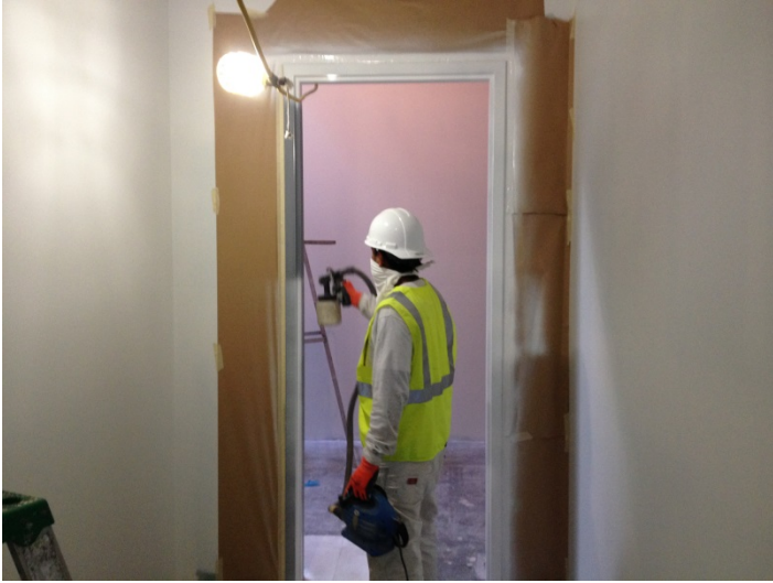
Date: 03/31/16 Quad County painting hollow metal door frames throughout the building.
