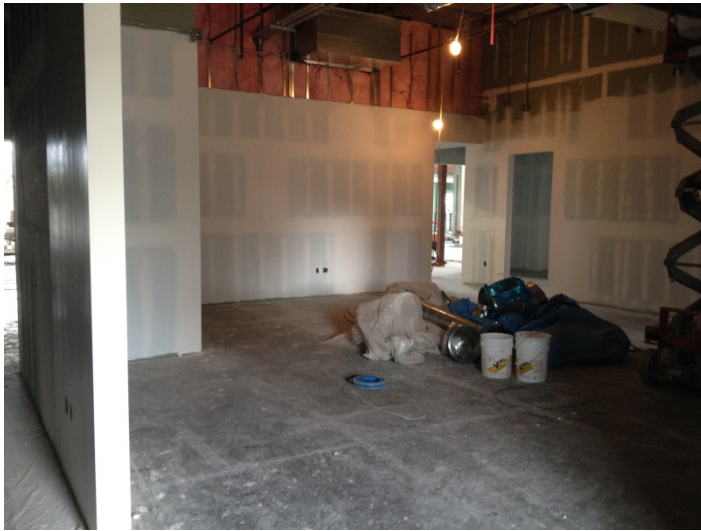
Date: 03/28/16 Painters onsite to prime interior walls. Picture depicts staff workroom.
