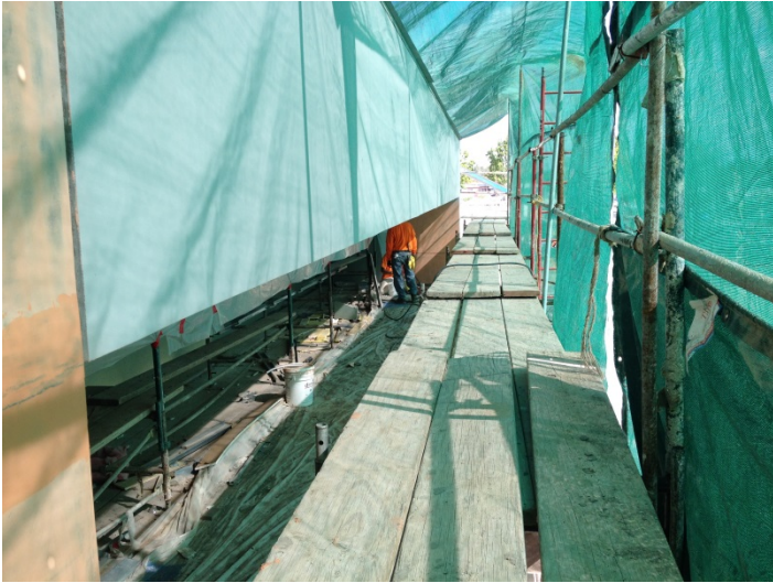
Date: 03/30/16 Rutherford priming EIFS along East elevation of community room.
