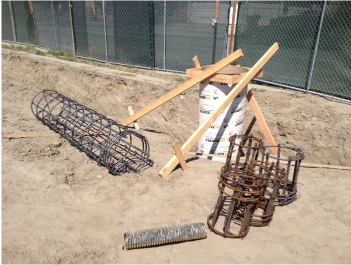
Date: 04/14/16 Rebar cages for light pole bases delivered to site.
