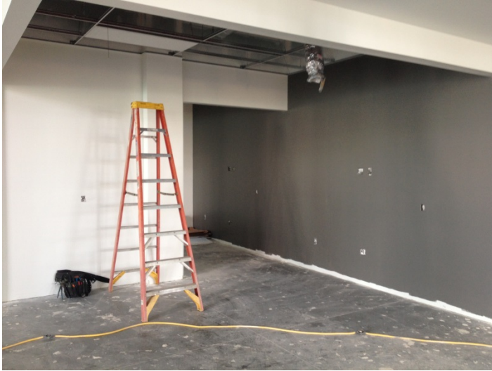
Date: 04/11/16 Painted walls located in Teen Study Rooms.
