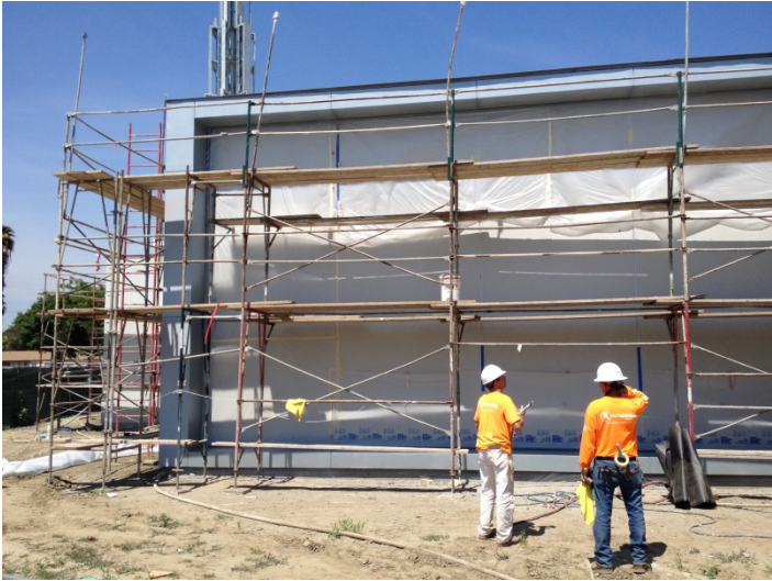
Date: 04/13/16 EIFS panels receiving final coating along Southern elevation.
