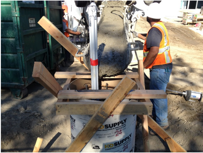
Date: 04/20/16 WCF onsite pouring concrete for light pole bases.
