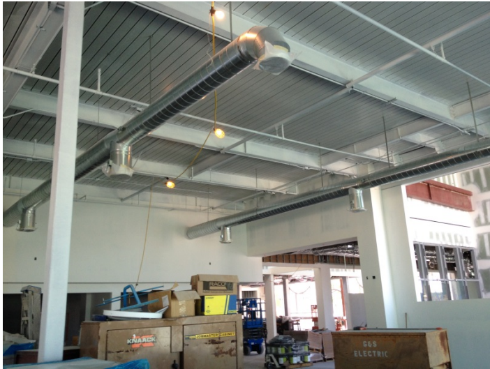
Date: 04/18/16 Quad County priming exposed beams in teen collection area.
