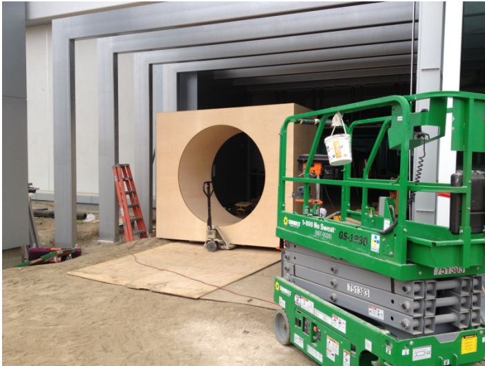
Date: 06/03/16 Children's collection circular entrance way being delivered to the site.
