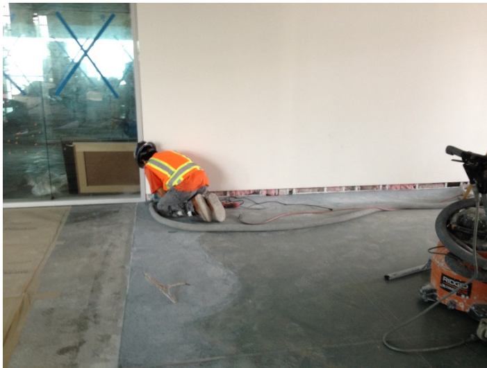
Date: 06/01/16 Continued grinding of epoxy terrazzo at lobby entrance to Library.
