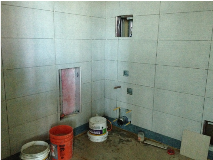
Date: 06/03/16 Installed wall tile in family restroom.
