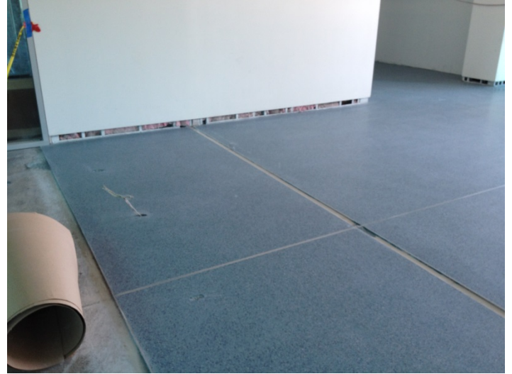
Date: 06/03/16 Progress of terrazzo at lobby entrance.
