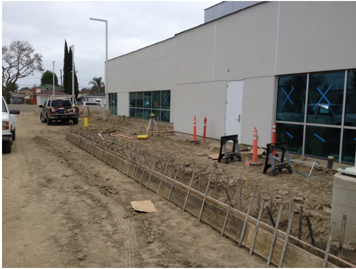
Date: 05/31/16 Curb formwork along the North end of the project site.
