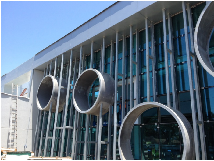
Date: 06/02/16 TMG continuing installation of glazing at West elevation fin wall.
