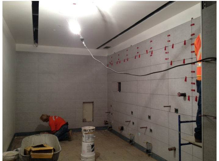
Date: 06/09/16 Progress of wall tile installation in men's restroom location.
