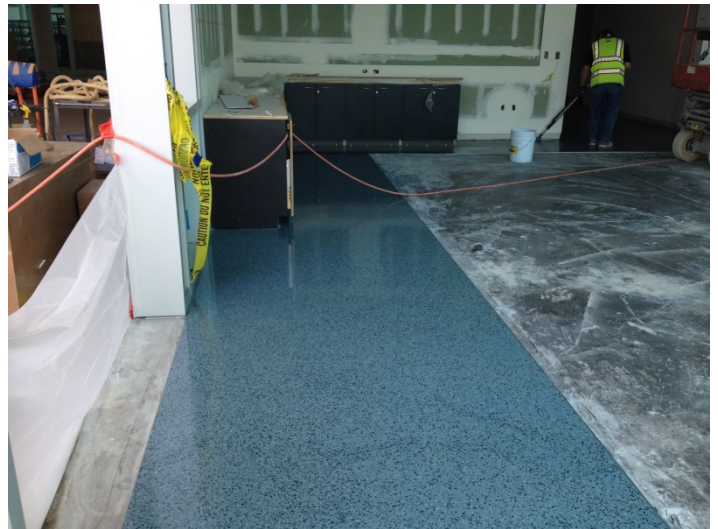
Date: 06/10/16 Sealer application to terrazzo in the large meeting room.
