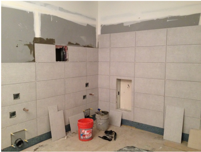
Date: 06/06/16 Installation of wall tile in the women's restroom.
