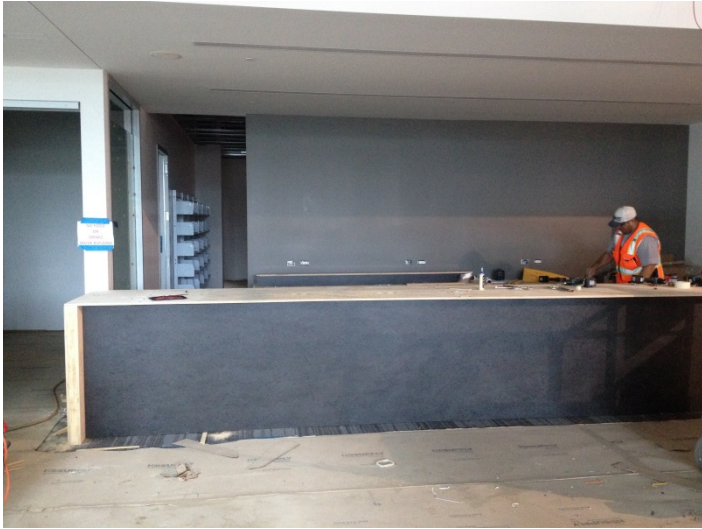
Date: 06/09/16 Progress of main circulation desk construction.
