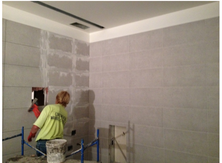
Date: 06/08/16 Corradini grouting wall tile in the women's restroom.
