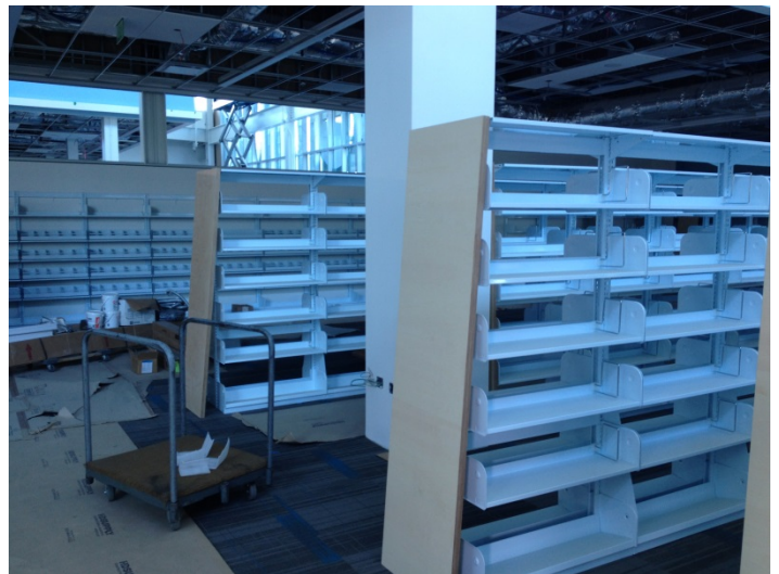
Date: 06/17/16 Layout for installation of end panels at stacks in the adult collection area.
