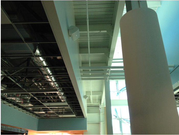
Date: 06/16/16 Speakers installed at soffit between children's and small children's collection area.
