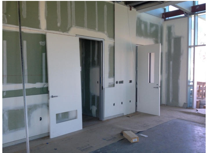
Date: 06/16/16 Additional door installation throughout the Library, doors lead to AV room and pantry from large community room.
