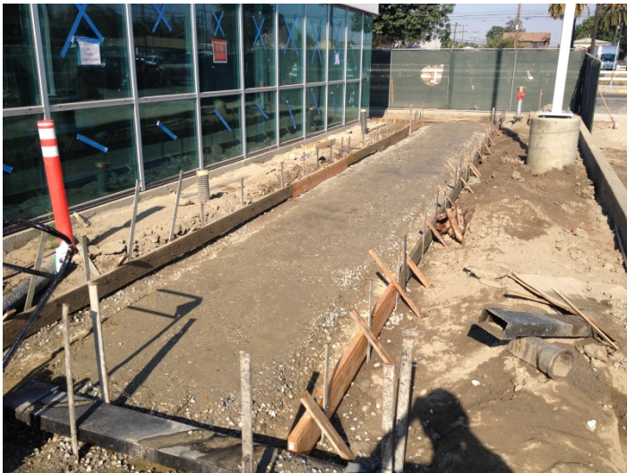
Date: 06/17/16 WCF starting to place aggregate base material at sidewalk locations around the perimeter of the site.
