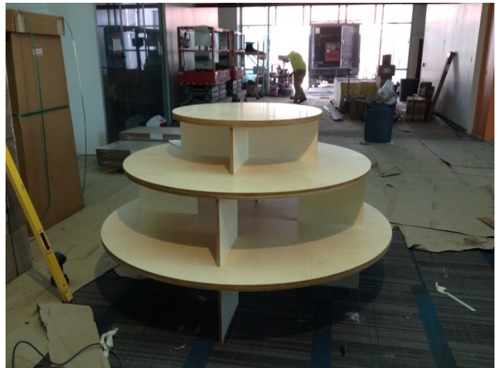
Date: 06/28/16 New book circular display table installed at entrance to the Library.
