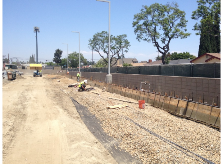
Date: 06/27/16 Progress of formwork for curb along Lime Avenue.
