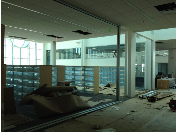
Date: 06/30/16 Installed framing for glazing at children's collection.
