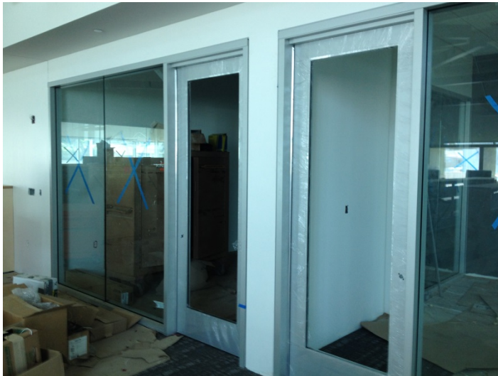
Date: 06/28/16 Installed doors at teen study rooms pending installation of glazing.
