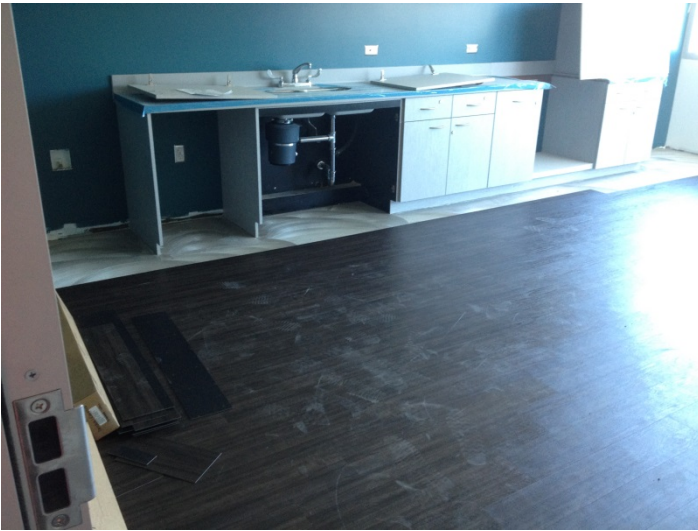
Date: 07/12/16 Resilient flooring installed in staff lounge.
