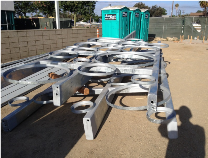
Date: 07/11/16 North bubble wall delivered to site.
