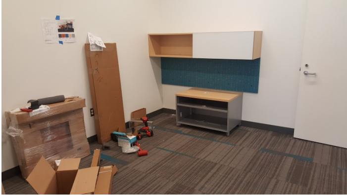
Date: 07/15/16 Progress of furniture installation in the manager's office.
