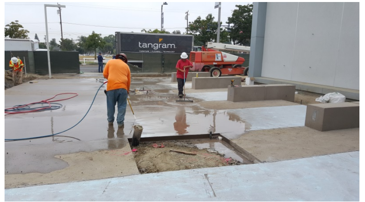
Date: 07/15/16 Top cast being power washed to expose aggregate of concrete walkway leading to Library entrance.
