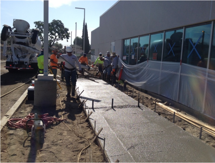
Date: 07/25/16 Concrete placement at sidewalk located at the North perimeter of the Library.
