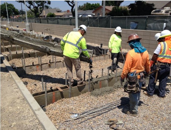
Date: 07/28/16 Concrete for curbs separating permeable pavement parking spots.
