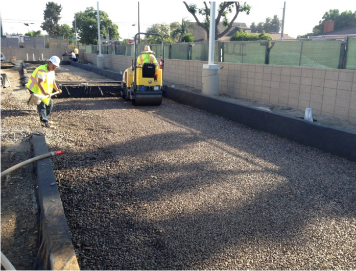
Date: 07/27/16 WCF installing ¾ -inch rock at permeable pavement.
