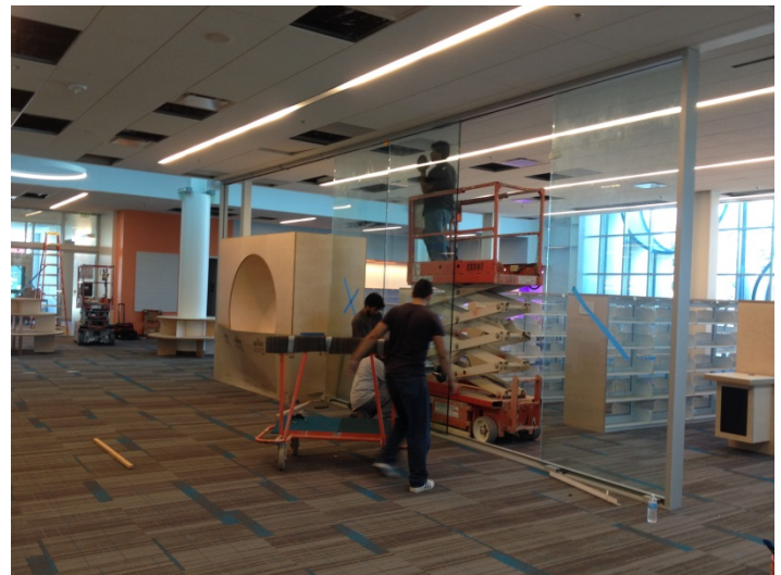
Date: 07/26/16 Glazing installation along entrance to children's collection adjacent to porthole entrance.
