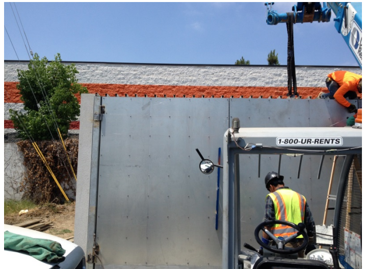
Date: 08/05/16 Bridge Iron onsite installing gate at trash enclosure.
