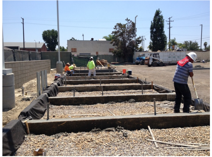
Date: 08/01/16 Site concrete contractors placing additional concrete at permeable parking stall curbs.
