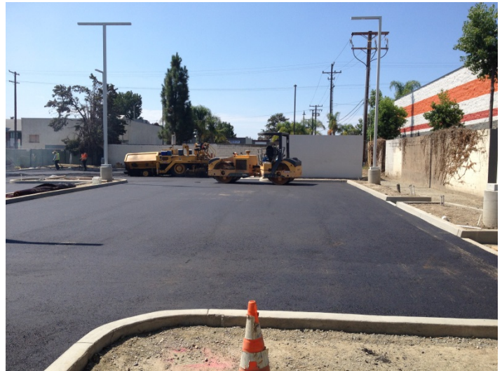
Date: 08/03/16 Progress of asphalt paving in the Southern parking lot area.
