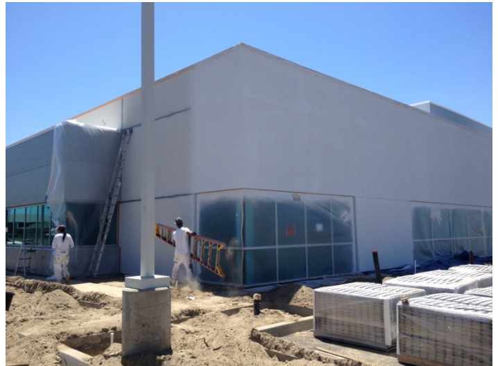
Date: 08/11/16 Progress of exterior plaster paint application at the Northeast corner of the building.
