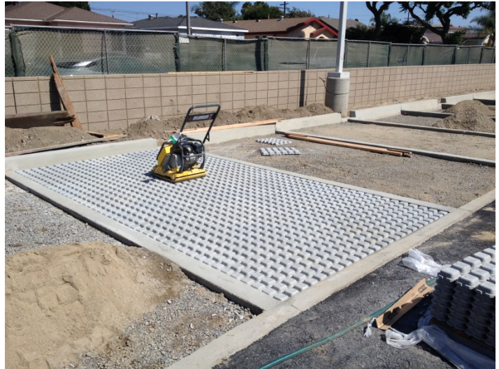
Date: 08/08/16 WCF installation of permeable pavement along the East end of the site.
