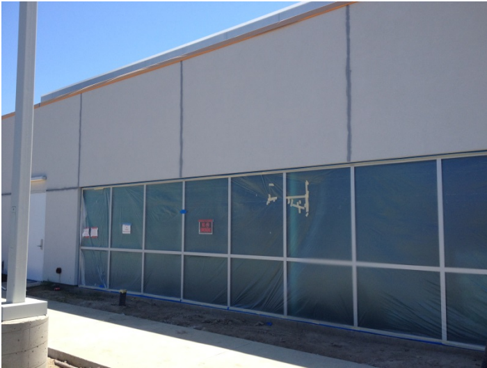
Date: 08/10/16 Painter masking glazing installed at the North elevation of the building in preparation for exterior paint.
