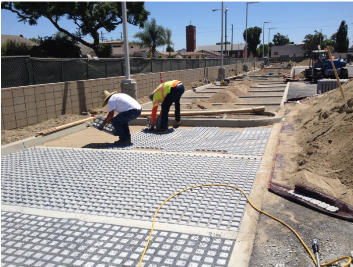
Date: 08/11/16 Progress of permeable pavement installation.
