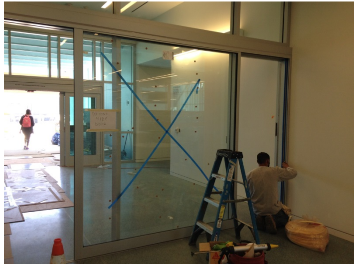
Date: 08/10/16 Glazer installing manual sliding door in Lobby area.
