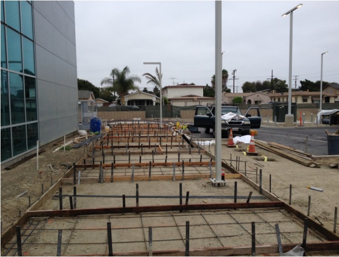
Date: 08/08/16 Site concrete subcontractor completing formwork and rebar installation for remaining paseo concrete.
