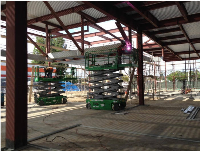
Date: 10/15/15 Bridge Iron welding trellis over entrance to the Library.
