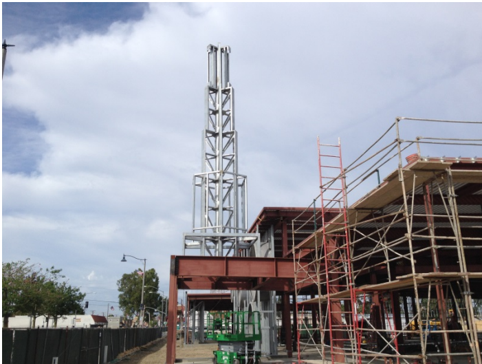
Date: 10/14/15 Erection of tower steel at the project site.
